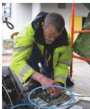
Manual wiring of junction box
